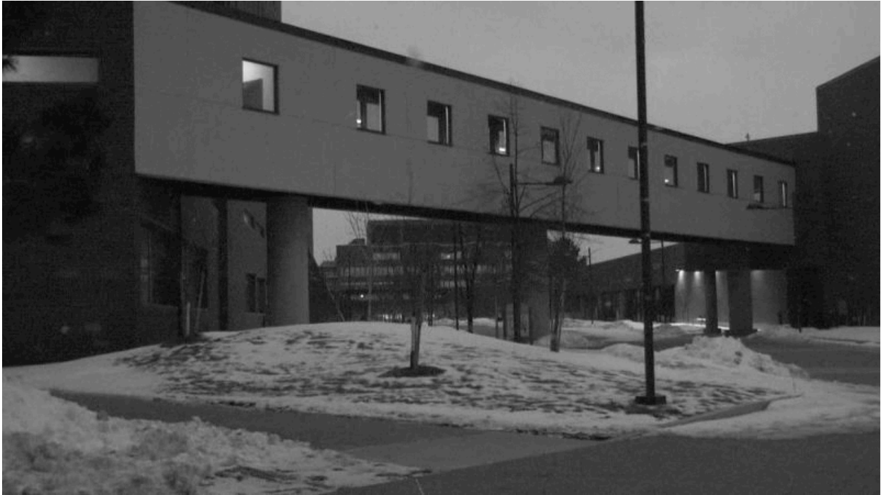
Figure 7: One of the 418 input images for the ‘Spines’ set of test images used in developing the project.
